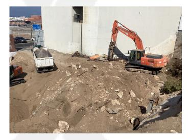
excavation required more time because of site condition and the nature of the difference between actual and proposed levels
